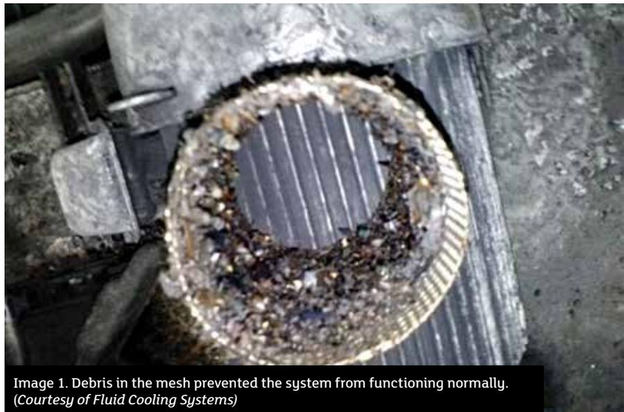
Image 1. Debris in the mesh prevented the system from functioning normally. (Courtesy of Fluid Cooling Systems)
