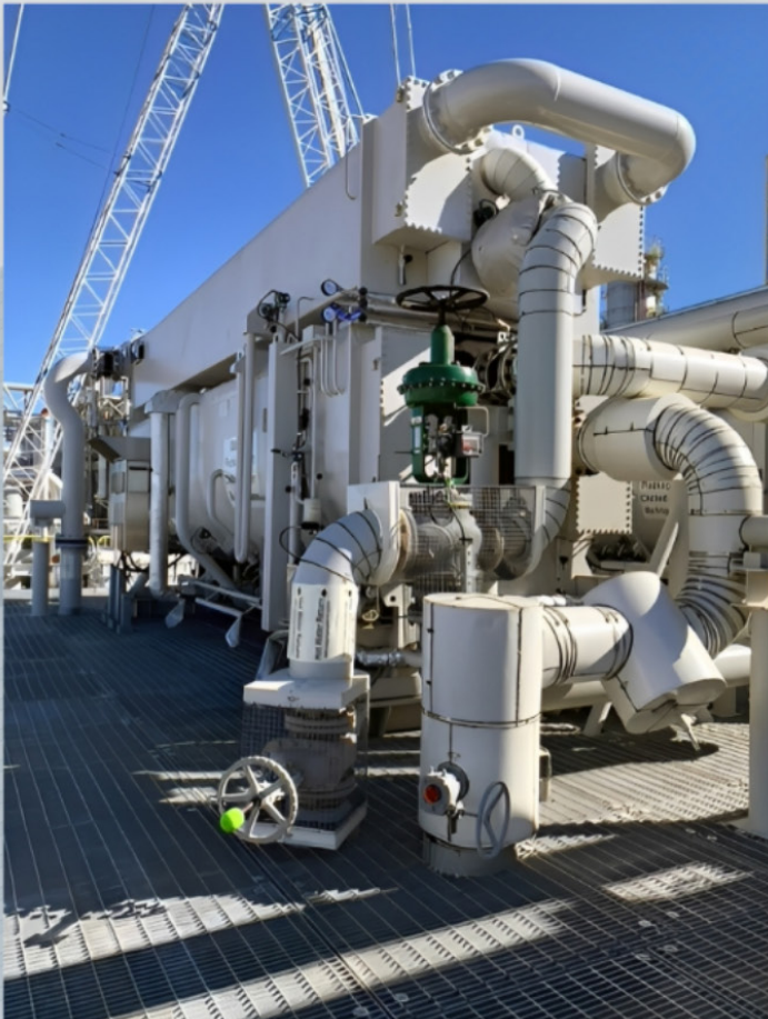
Shuangliang absorption chillers. Steam, gas fired and heat pumps are available.
